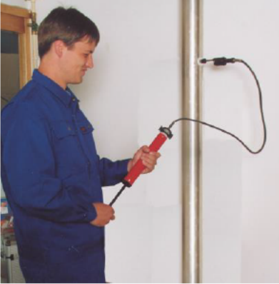
Fig. 4: Extracting the smoke gas
