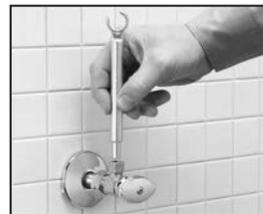
The lug at the end of the smaller wrench is inserted into the riser mouth of the angle stop for pointing and stability. Point it at the optimum angle for later insertion of the supply tube...
