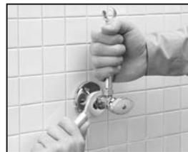
...the larger wrench is then used to tighten the back compression nut.
