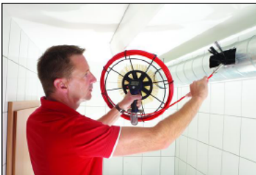
Fig. 21: Cleaning a ventilation duct
