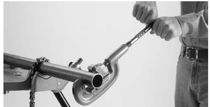
Figure 3 – Cutting End Of Pipe
