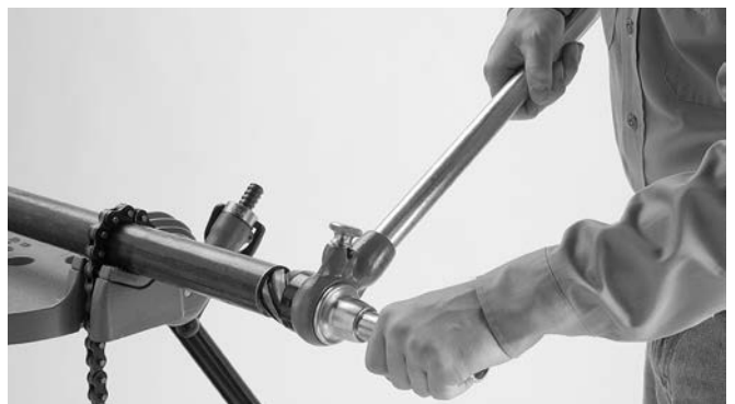
Figure 4 – Reaming End Of Pipe
