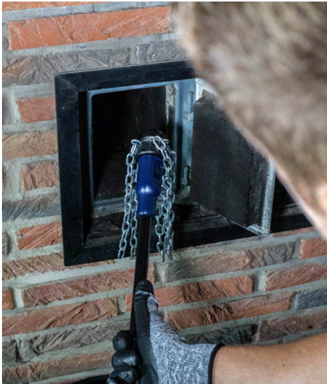
The universal rotary head can be equipped with chains. So even persistent soot is no longer a problem for you.
