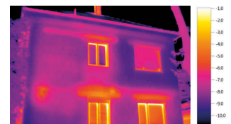
Thermal image with ScaleAssist
