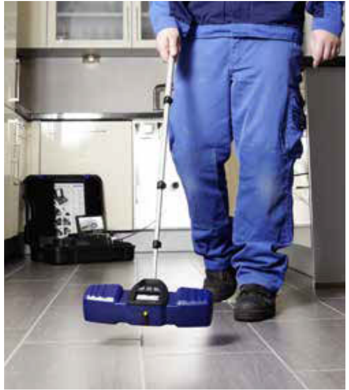
The actual meter count and the position of the head are displayed in the monitor. The Wohler L 200 Locator makes it possible to locate the camera.
