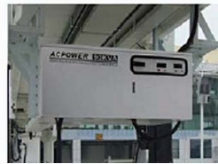
Airport Apron / Hangar
