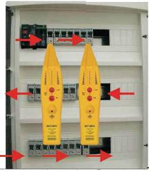
The Circuit breaker which supply the Transmitter circuitry is the one, which, when pointed out by the tip, has the most LEDs lit on the bar-graph and the fastest buzz.
