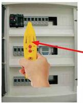
The Bar-Graph shows that the first circuit breaker of the first row has no signal on it. It buzz very slow too. The battery voltage is ok. You can go left and right and change row as you want to.
