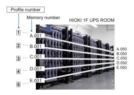
You can save measured data associating with profile information previously registered. This makes the control of information, including the UPSs equipped with batteries under measurement and their locations, easier.
