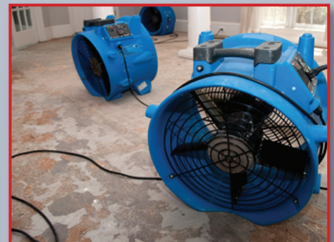
Air movers wrapping up a water damage restoration project
