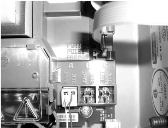
Fig. 11. Sensor Polarity. When current sensor is installed properly, error LED is off. If the Error LED is illuminated, then disconnect the gray plug and reverse the input lead. If it clears, the “Sensor Error” then mark appropriately. Repeat for all sensors.
