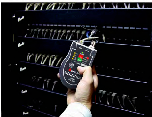
Confirm continuity and fault type
