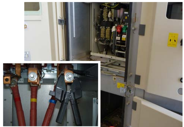
DLRO100 testing circuit breaker
