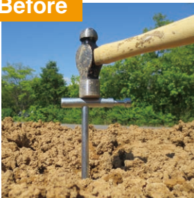
Thick rods had to be hammered into the ground and were difficult to remove.
