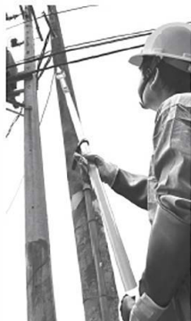
Fig. 3: Voltage detection for overhead lines
