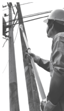
Fig. 3: Voltage detection for overhead lines
