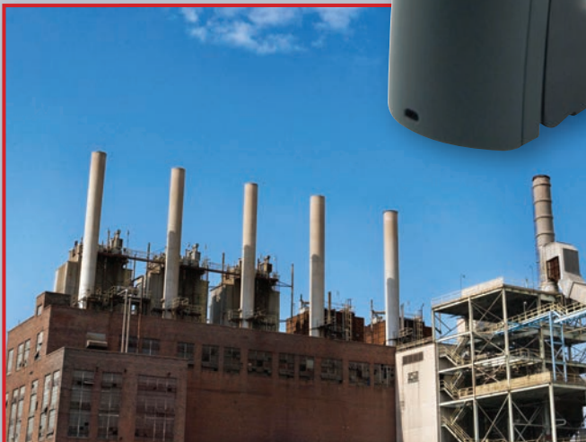
Industrial site inspection
