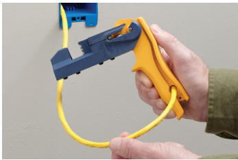
1. Strip cable jacket with a standard cable stripper or the built-in cable stripper.
