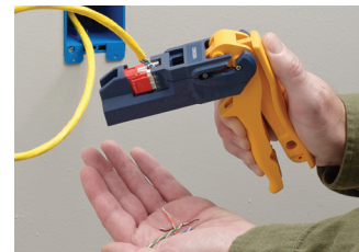
6. Wires will be seated and cut for a solid termination.
