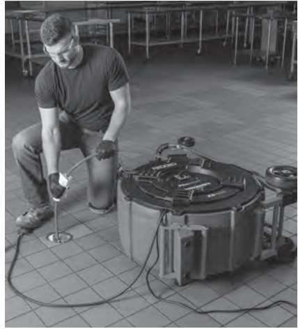
Figure 9 – Applying Lubricant to the Cable Sheath
