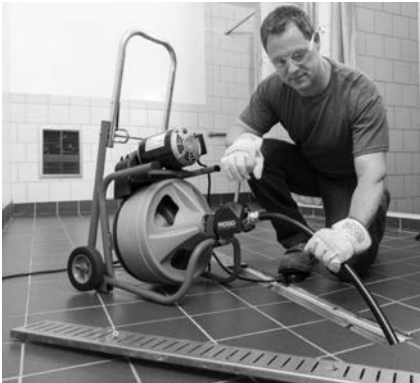
Figure 16 – Using Machine with Guide Hose
