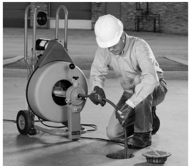
Figure 12 – In Operating Position, Manually Feeding Cable
