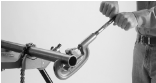
Figure 1 – Cutting End of Pipe
