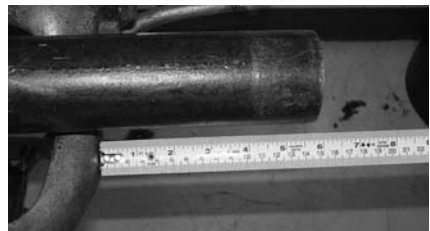
Figure 9 – Pipe in 300 Power Drive, Inspecting for Prep Tool Adequate Clearance
