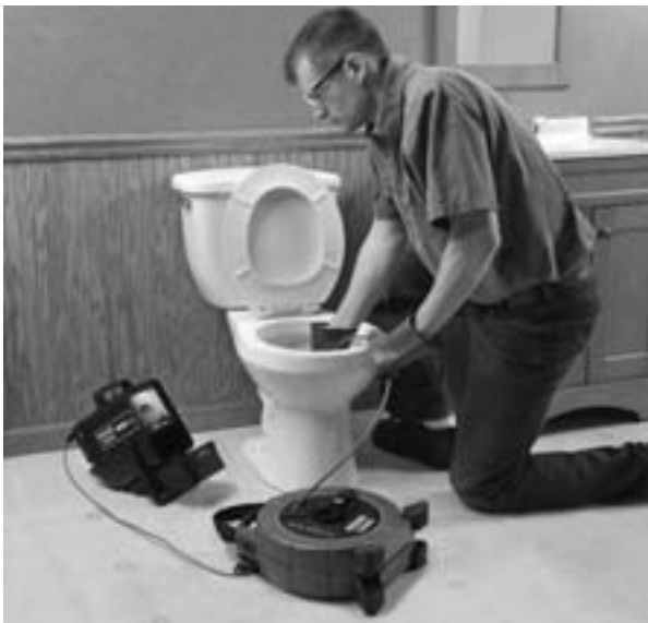
Figure 15 – Doing An Inspection
