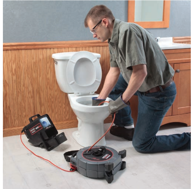
Figure 14 – Performing an Inspection
