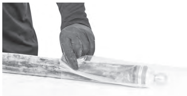
Figure 12 – Inserting Packer Into Sleeve
