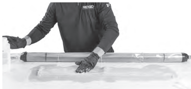
Figure 28 – Wetting Out The Patch Off The Packer
