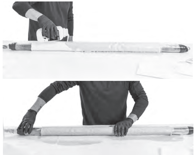
Figure 33 – Wetting Out The Patch On The Packer
