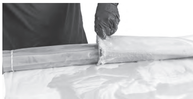
Figure 29 – Inserting The Packer In Patch
