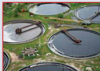
Water Pollution Control
