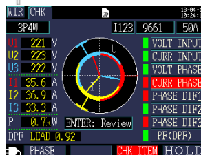
Wiring Check screen
