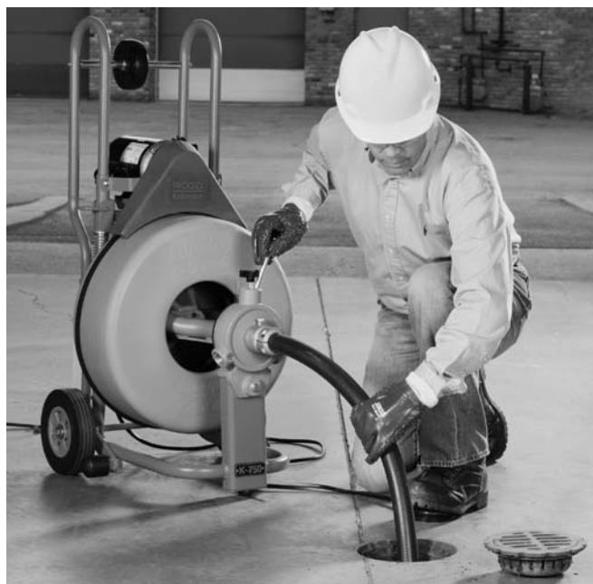
Figure 15 – Using Machine with Guide Hose
