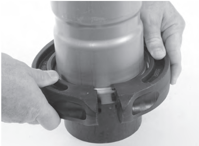
Figure 11 – Installing Press Ring Onto Fitting
