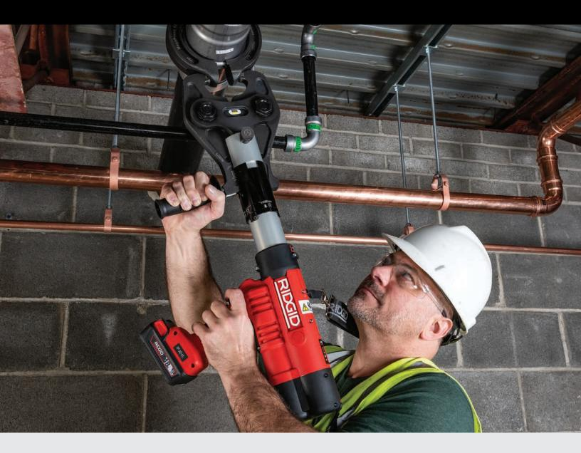
The RP 342-XL is the first ever RIDGID<sup>®</sup> press tool that works on any size and material pipe. From ½" PEX all the way up to 4" carbon steel\*, one tool can press it all. It also works with the full line of RIDGID Standard 32kN attachments including fan favorites like StrutSlayr<sup>®</sup> and PressSnap<sup>®</sup>. Its compact design and versatile applications make it the tool you want for every job.
