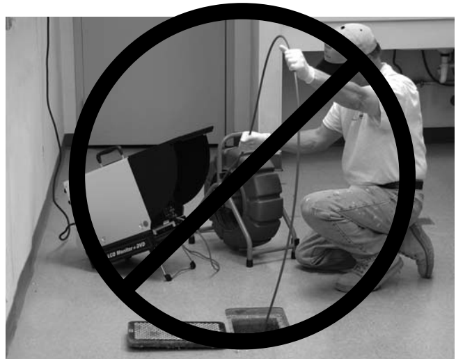
Figure 27 – Improper Cable Push
