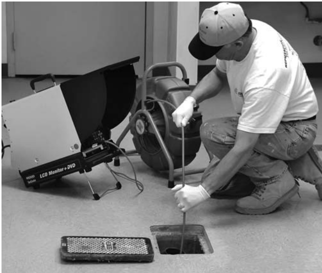
Figure 28 – Proper Cable Push
