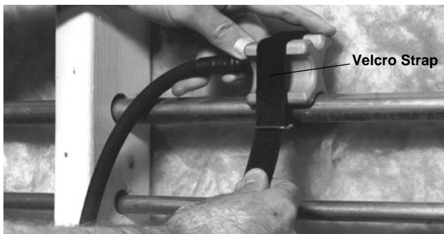
Figure 5 – Applying Freeze Head with Velcro Strap
