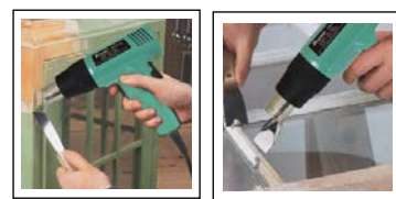
Paint and varnish removal
