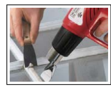
Removal of window glazing
