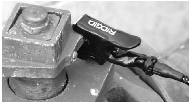
Figure 8 – Connecting Cable Lead To Target Conductor.
