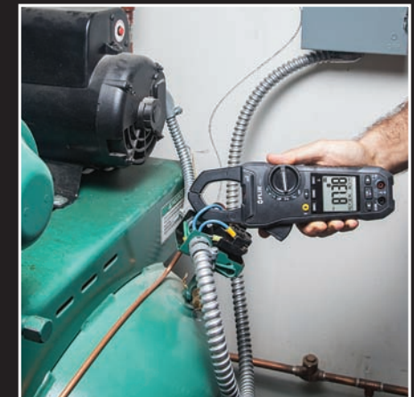
Inrush Current detects start-up current spikes
