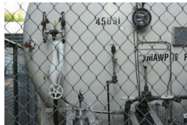
Difficult inspection sites
