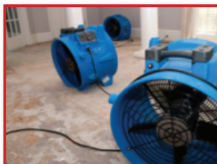
Monitor the drying part of water damage restoration
