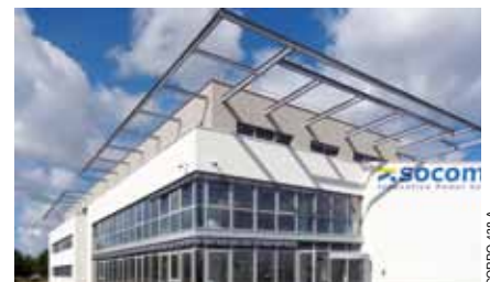
Socomec Green Building.
