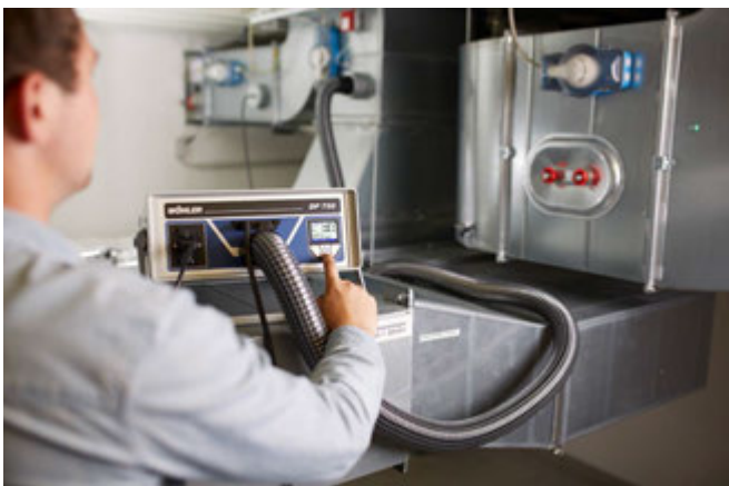
Leakage tests on several 100 m 2 of installed ductwork systems.
