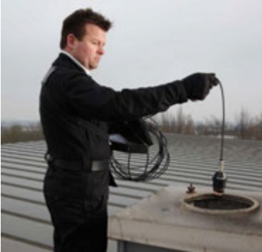
Fig. 5: Inspections using camera cable from above
